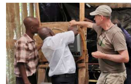
Installation of the soil moisture sensor for the Agro PV project
